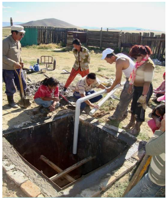
Project beneficiaries are installing ventilation channel for cellar.
